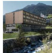
The JUFA-Hotel Grava with 80 rooms and 200 beds will be opening in the summer in Savognin. The special feature of the new accommodation: it consists mostly of QUADRIN-wooden modules by the local company Uffer AG. The ready-assembled and equipped hotel rooms just needed to be placed on top of and next to each other on the construction site with a crane.
